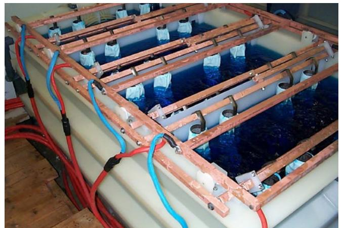
Figure 2: Acid copper electrolytic plating tank with excellent cable attachments from the rectifier to the bus bars, and multiple connections employed to improve current flow.
