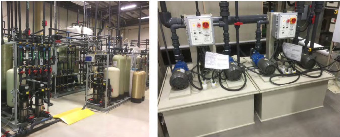
Figure 4: Key recovery systems of ion exchange, evaporation, crystallization, reverse osmosis, and electrolytic copper and tin electrowinning.
